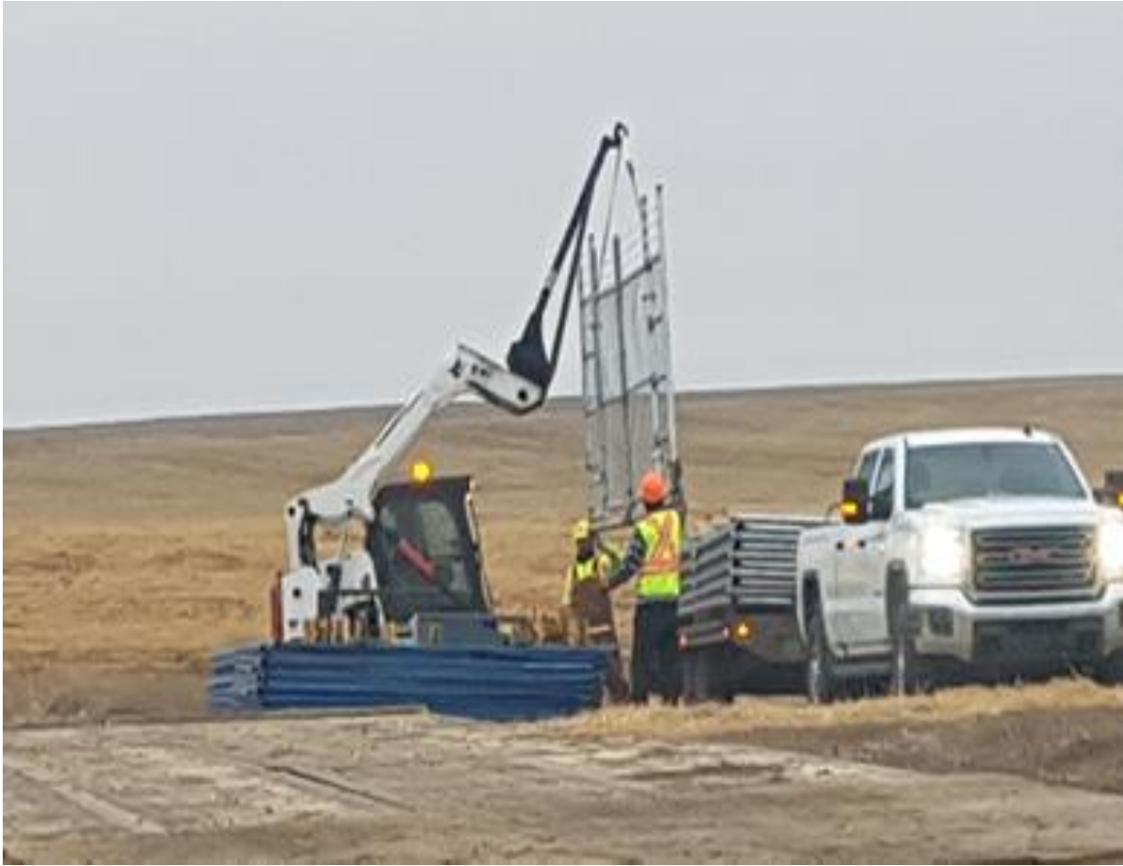
Unloading steel fence that is to be used as permanent fence around valve.
