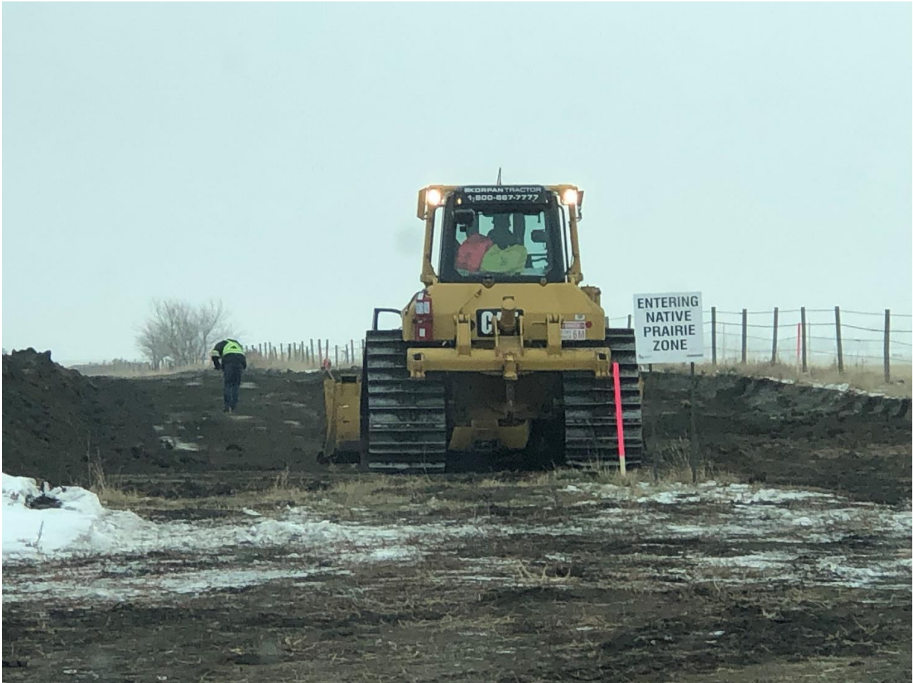
Grading access road so it is level.
