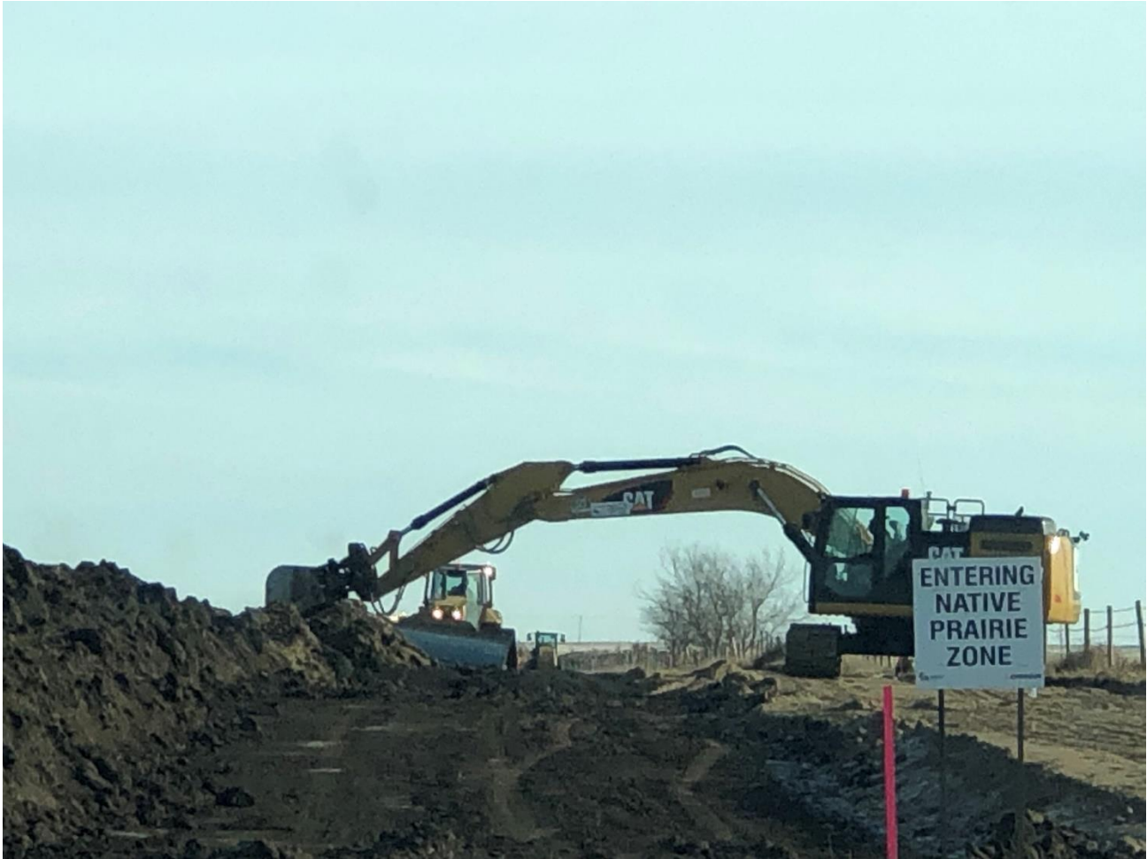
Stripping top soil at access road in Bethune pipe yard.
