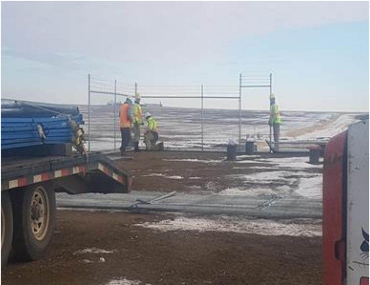
Assembling fence around pipeline valve.
